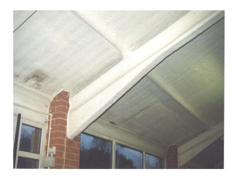
• Insulating boards used for fire protection, thermal insulation, partitioning and ducts.
